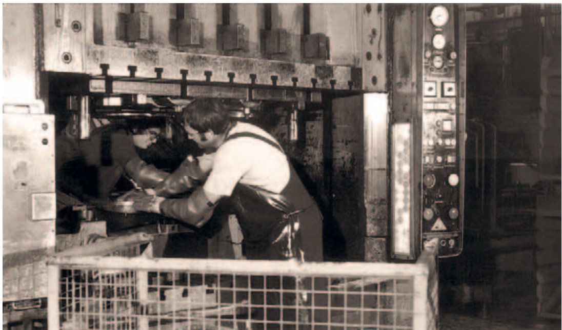
Fig. 19 Setting up work on an eccentric press: in the 1950s a focus of accidents continued to be the numerous serious accidents on presses. The precision engineering and electrotechnical Berufsgenossenschaft BG FE tried to inject fresh impetus into this area with the help of its own design office for press protection. Metal employer’s liability insurance associations joined in with this initiative.
